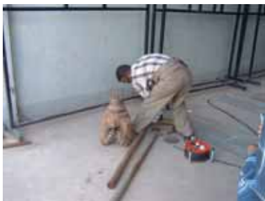
Above: Cutting work of wasted pipes
