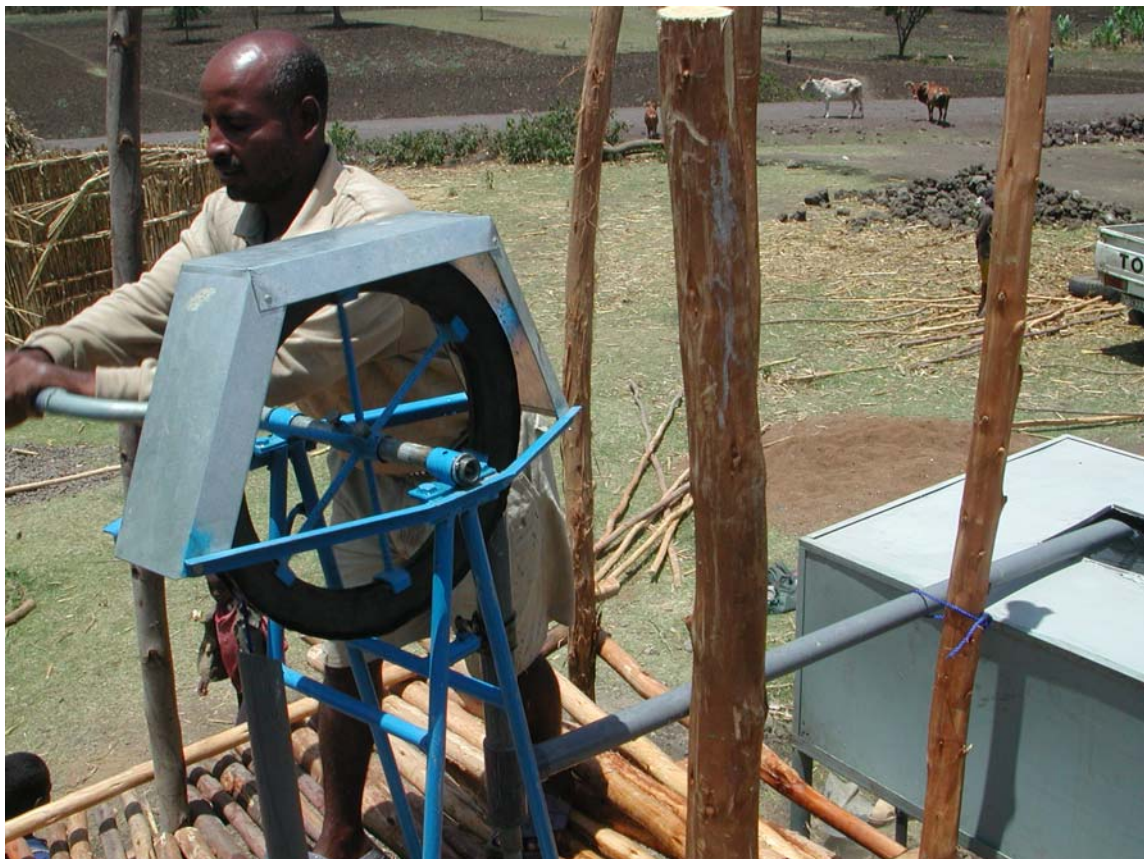
Photo 15. The owner of the well pumping using the installed rope pump
