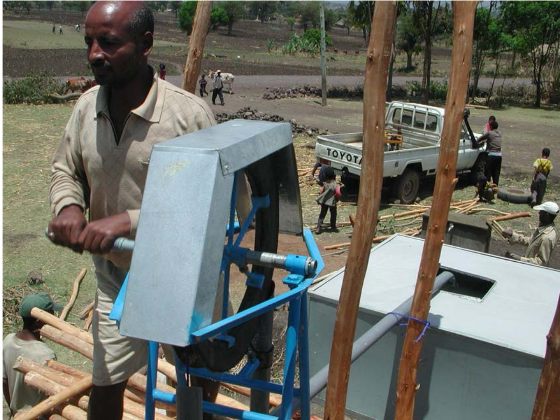
Photo 14. The owner of the well pumping using the installed rope pump
