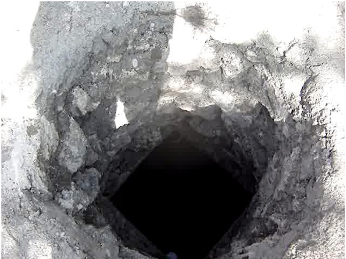
Photo 9. View of the hand dug well of Ato Bulema before installation of rope pump
