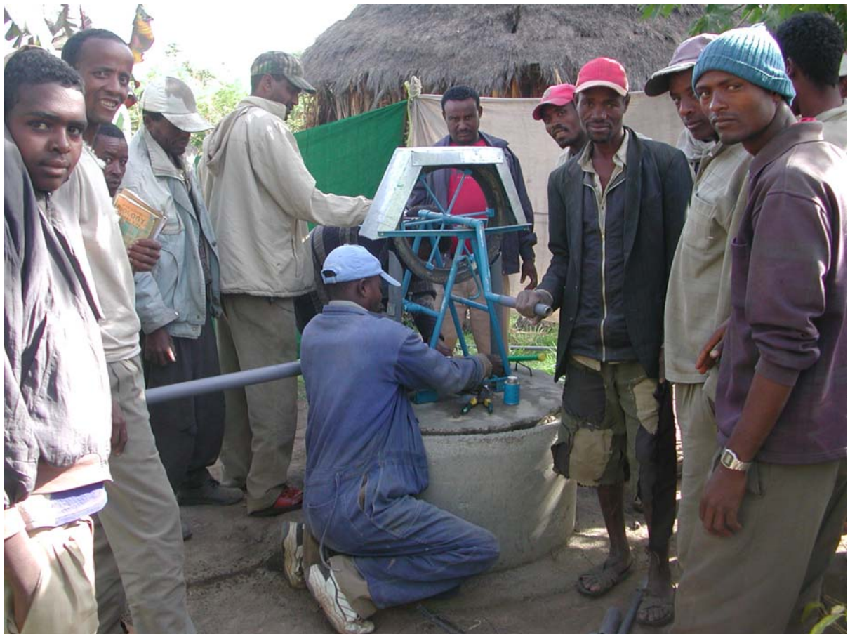
Photo 11. Installation of Rope pump at Ato Bulema dug well
