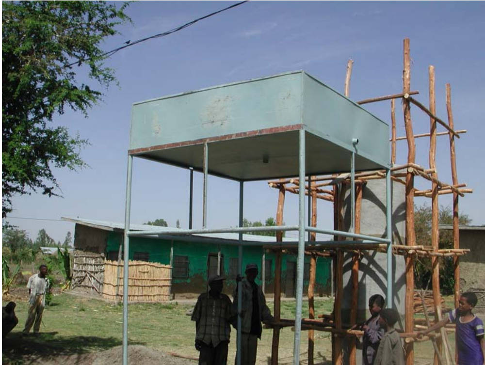
Photo 3. 2m 3 steel elevated tanker constructed at Kuno Kertafa
