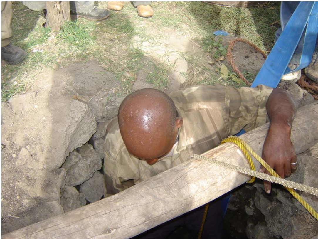
Photo 12. The owner of the well entering the well for deepening its depth
