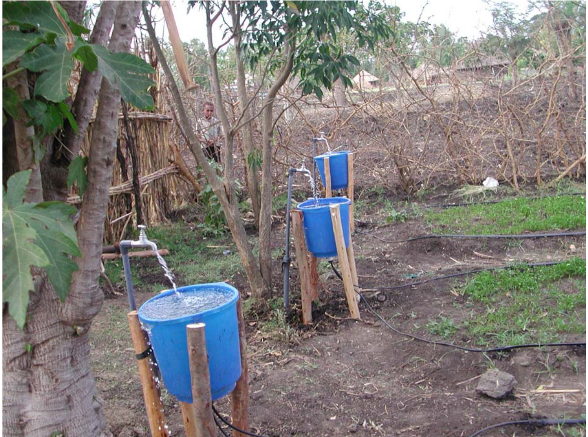
Photo 17. Drip irrigation installed at Dobena Bati
