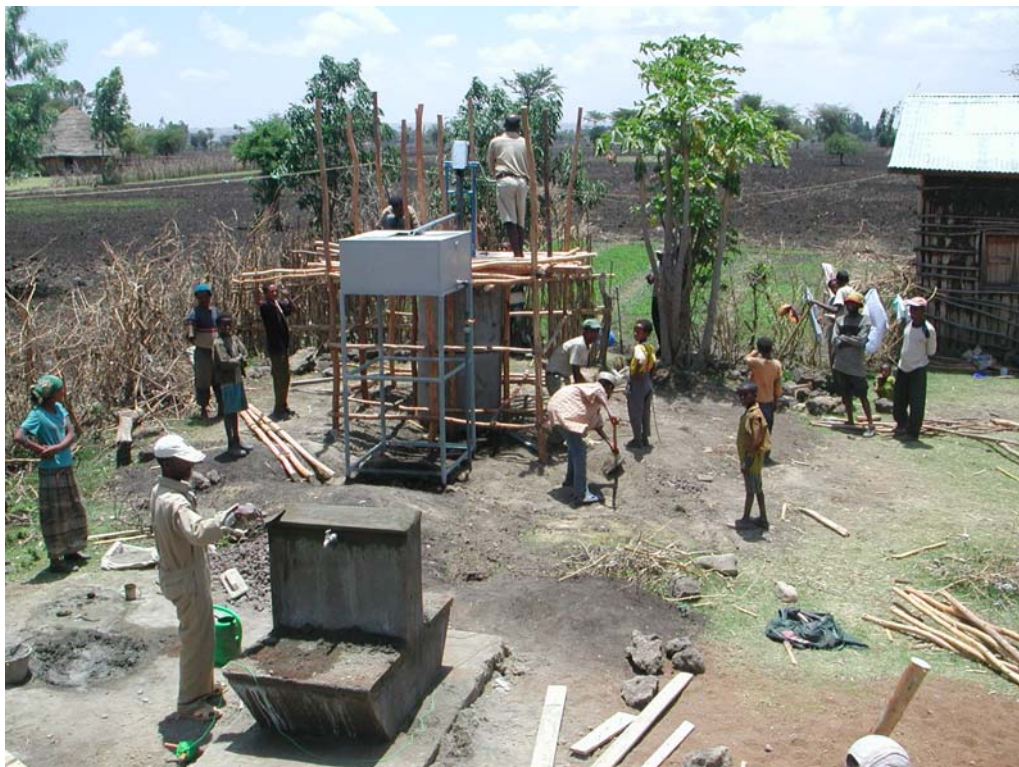
Photo 14. Construction of Dobena Bati community water supply with common rope pump
