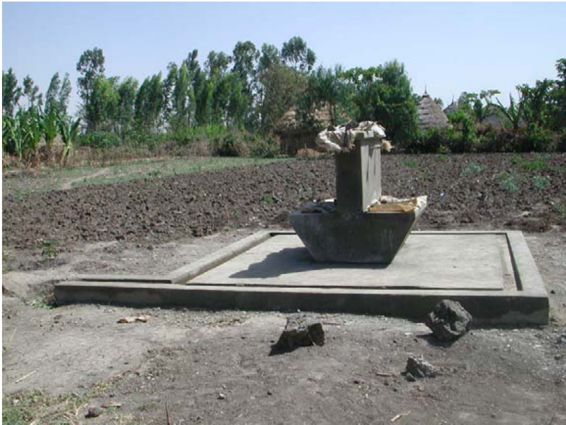
Photo 1, Constructed Public Fountain at Kuno Kertafa
