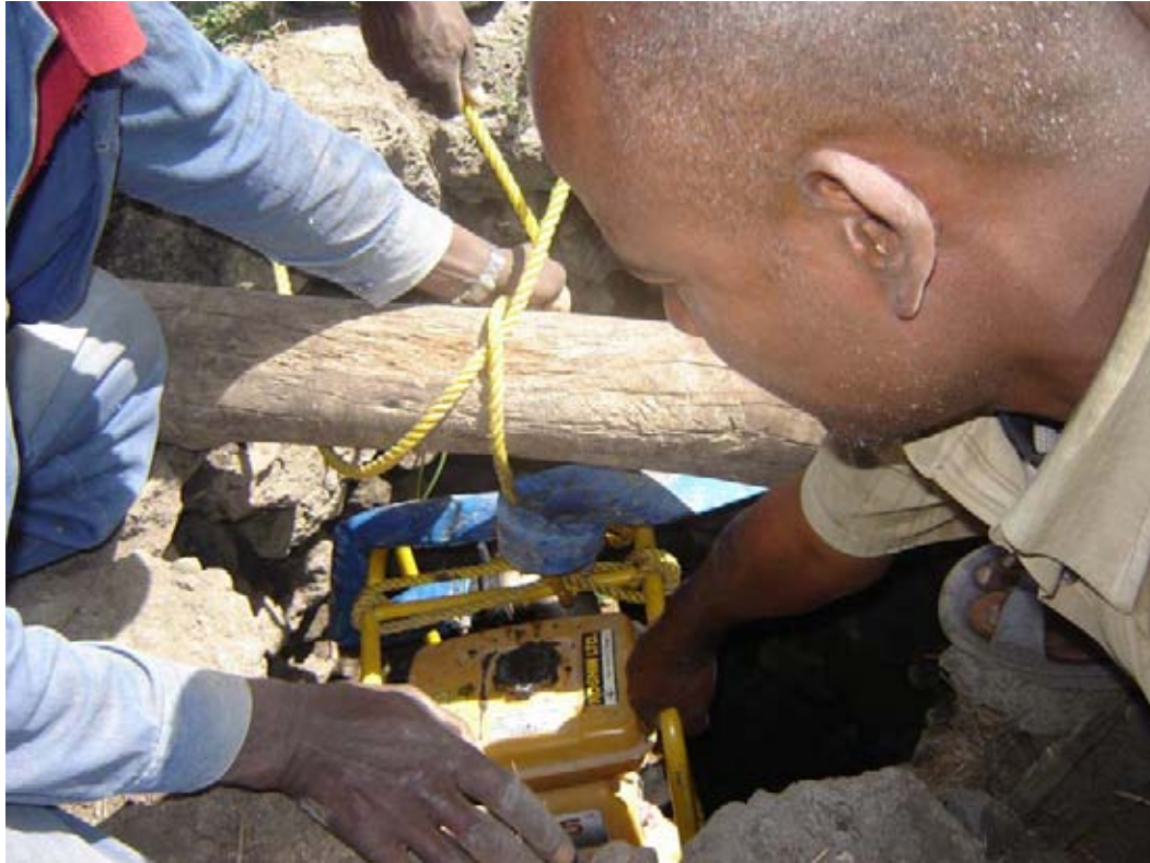
Photo 13. Removing dewatering pump after unsuccessful trial
