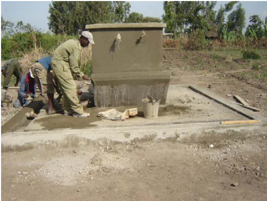
Photo 2. Construction of Public Fountain At Kuno Kertafa
